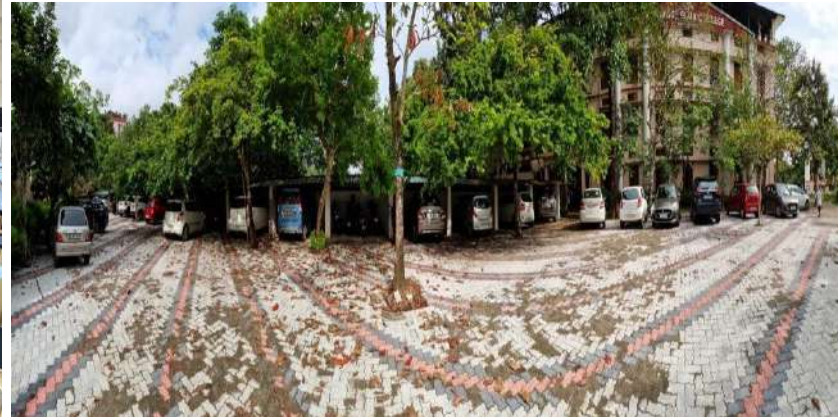
Renovated Parking Space
