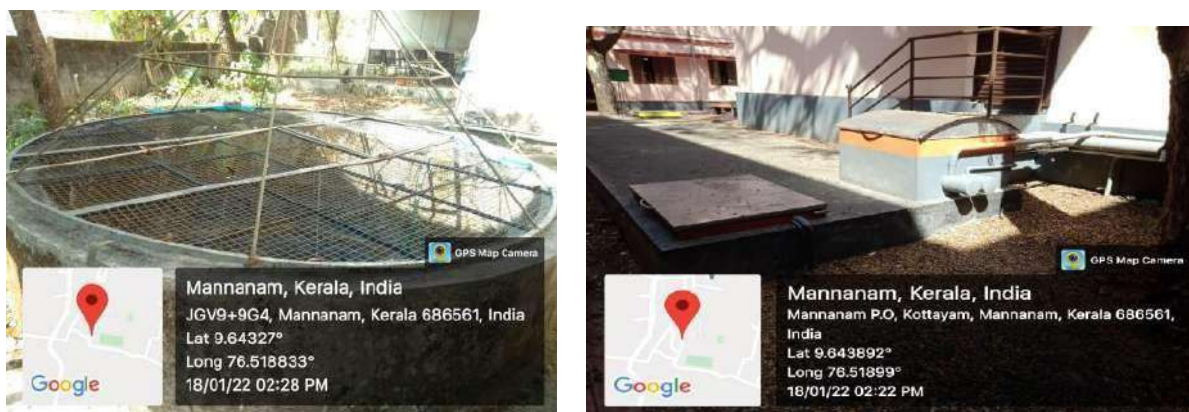
Fig. 10 Rain water harvesting structures
